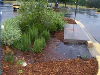
Stormwater collection islands provide an alternative way of dealing with storm water runoff.
