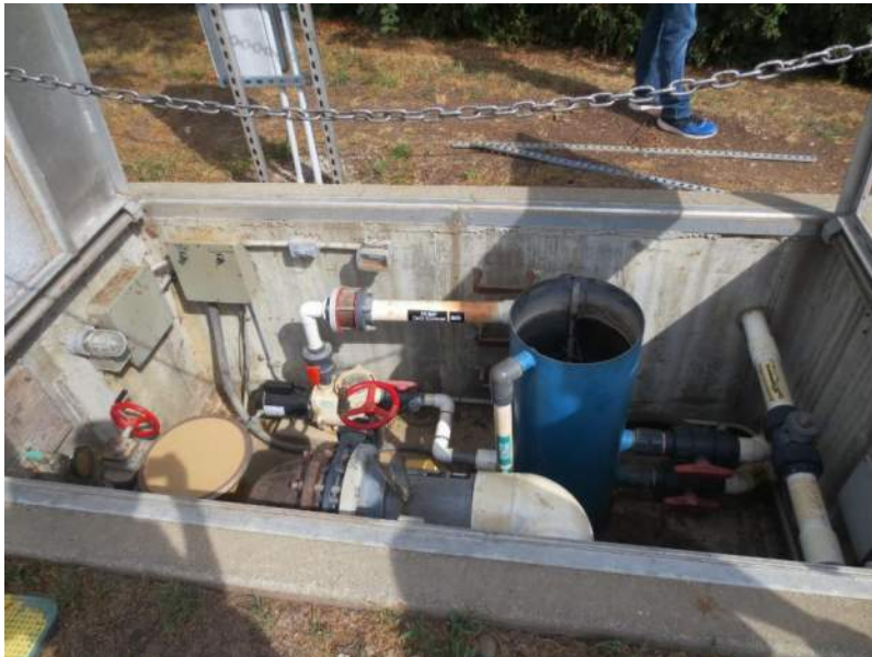
Flow Control Pit for Water Slides
