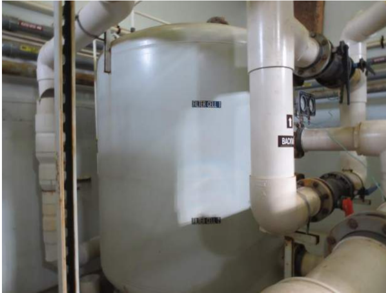
Dual Cell Filter (one of two)
