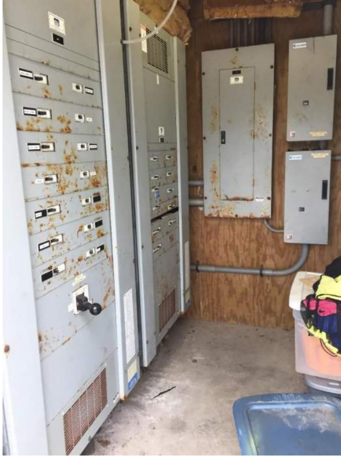
Electrical Control Room (note corrosion)
