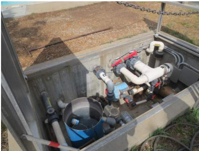
Vortex Pool Flow Control Pit
