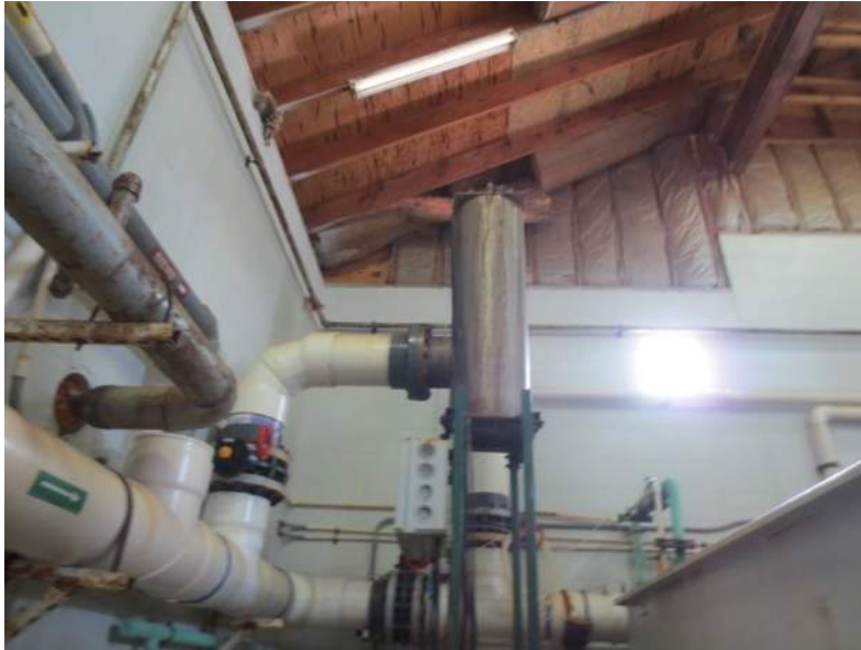
UV Unit and Balance Tank
