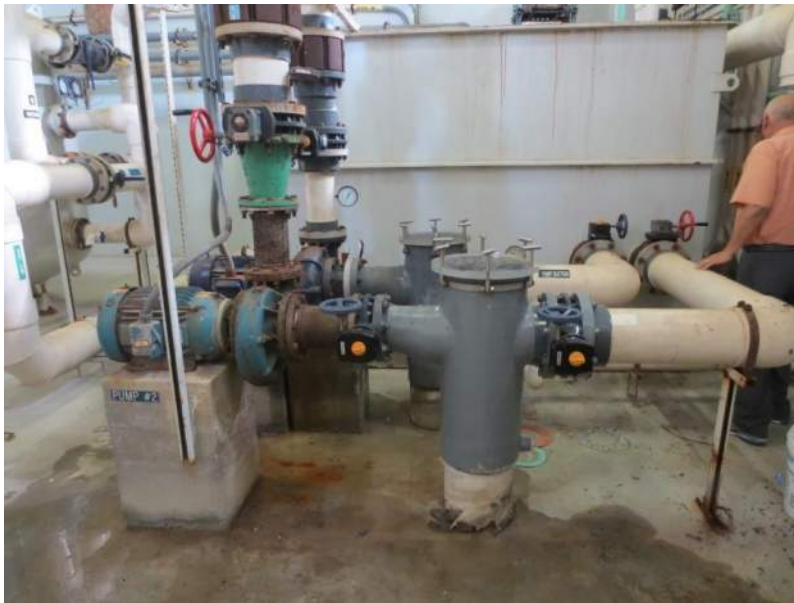
Main Recirculation Pumps, Strainers and Valves
