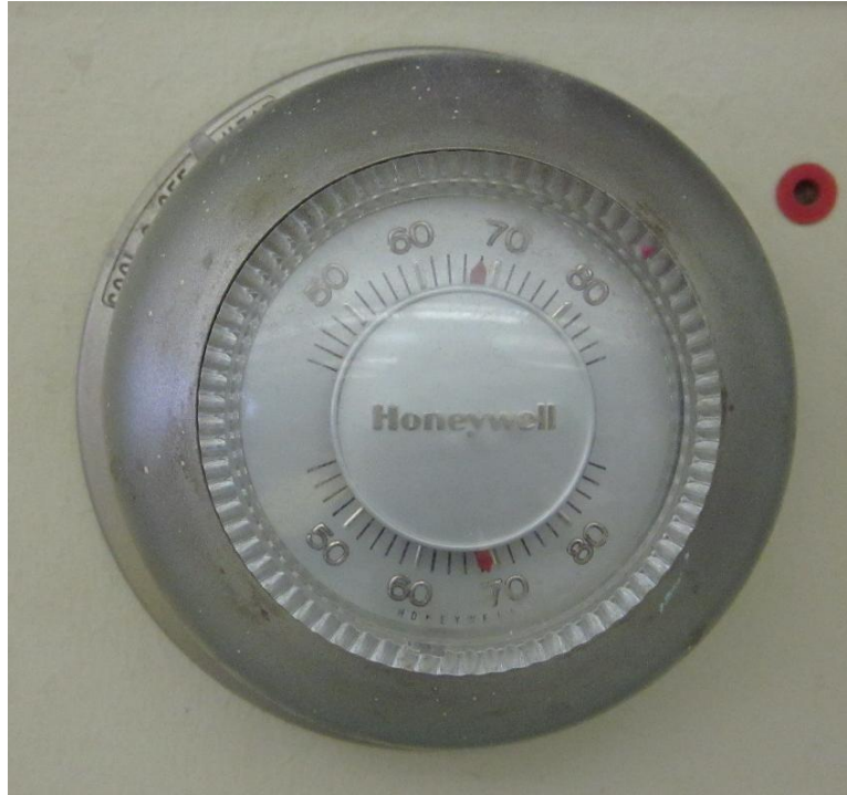
Figure 4.11.C: Typical Non-Programmable Thermostat
