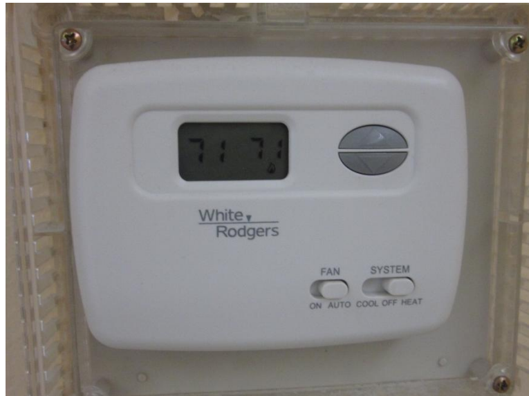
Figure 4.11.A: Typical Non-Programmable Split System Thermostat
