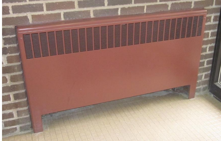
Figure 4.9.A: Typical Fan Coil Unit
