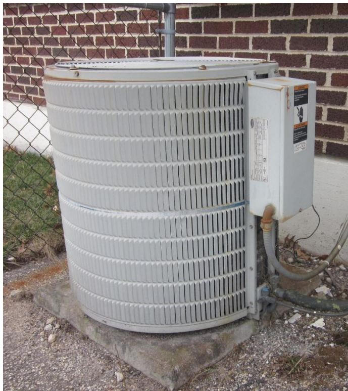
Figure 4.9.B: Typical Carrier Condensing Unit
