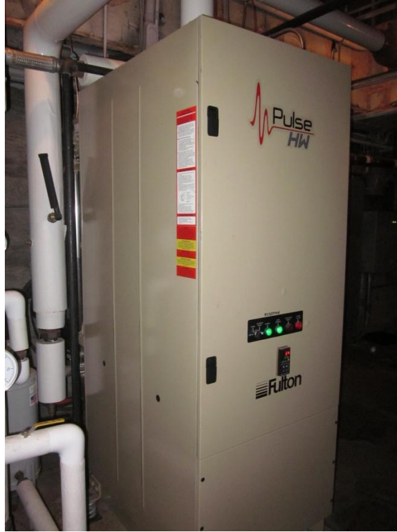
Figure 4.7.A: Community Center Condensing Boiler
