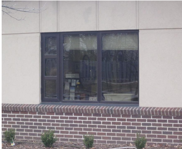
Figure 4.6.B: Typical Double Pane Window
