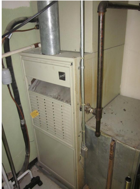
Figure 4.9.C: Typical Carrier Vertical Air Handler
