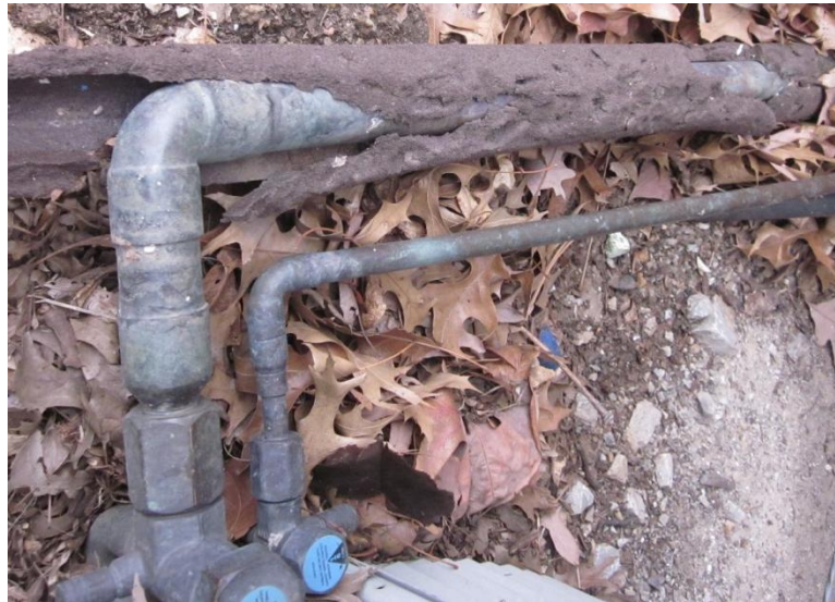
Figure 4.9.D: Typical Damaged Refrigerant Pipe Insulation
