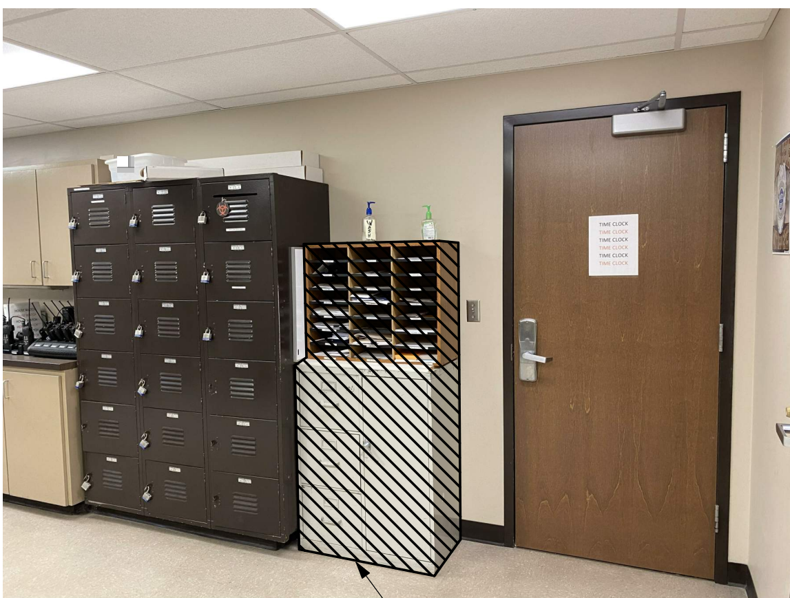
— REMOVE FILE CABINET TO COMPLY WITH ADA SECTION 404.2.4.1
