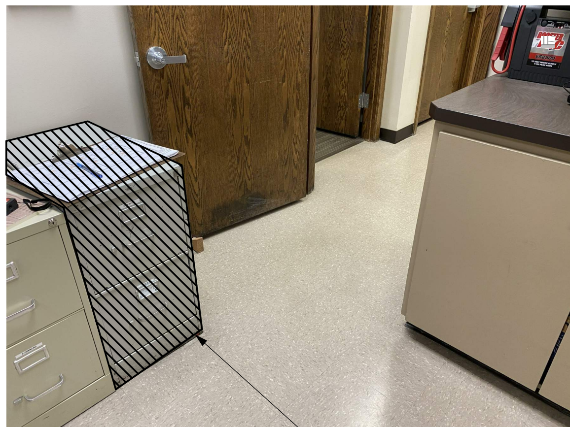
– REMOVE FILE CABINET TO COMPLY WITH ADA SECTION 403.5.1.
