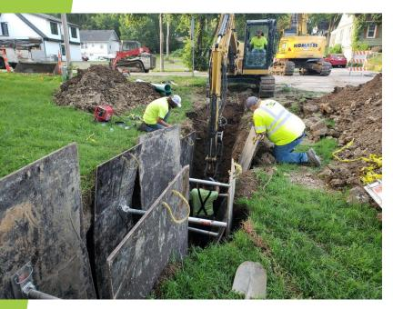
Contractor currently completing sanitary encasements and removal/installation of storm pipe between Roe Lane/Fontana
