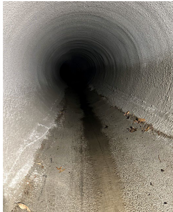
Concrete Lining Added
